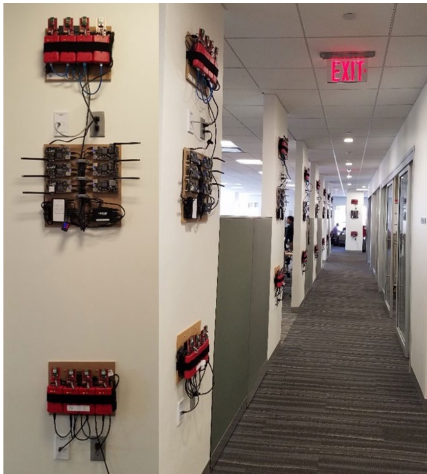
Figure 3-5 Testing Clusters in the Silicon Labs R&D Facility
